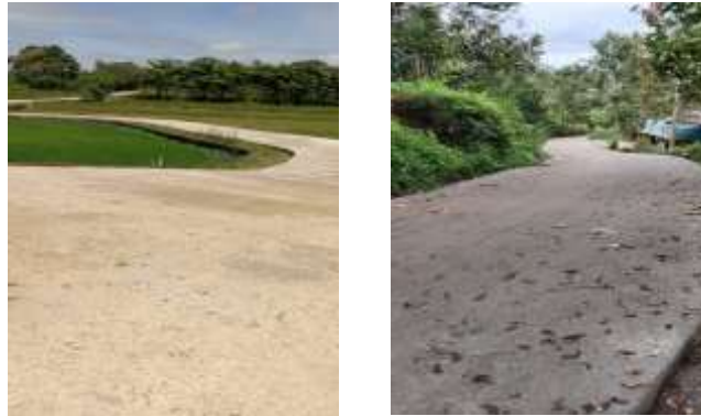
Figure 2 Road Construction and Repair
