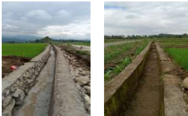
Figure 3 Construction of Irrigation Channels
